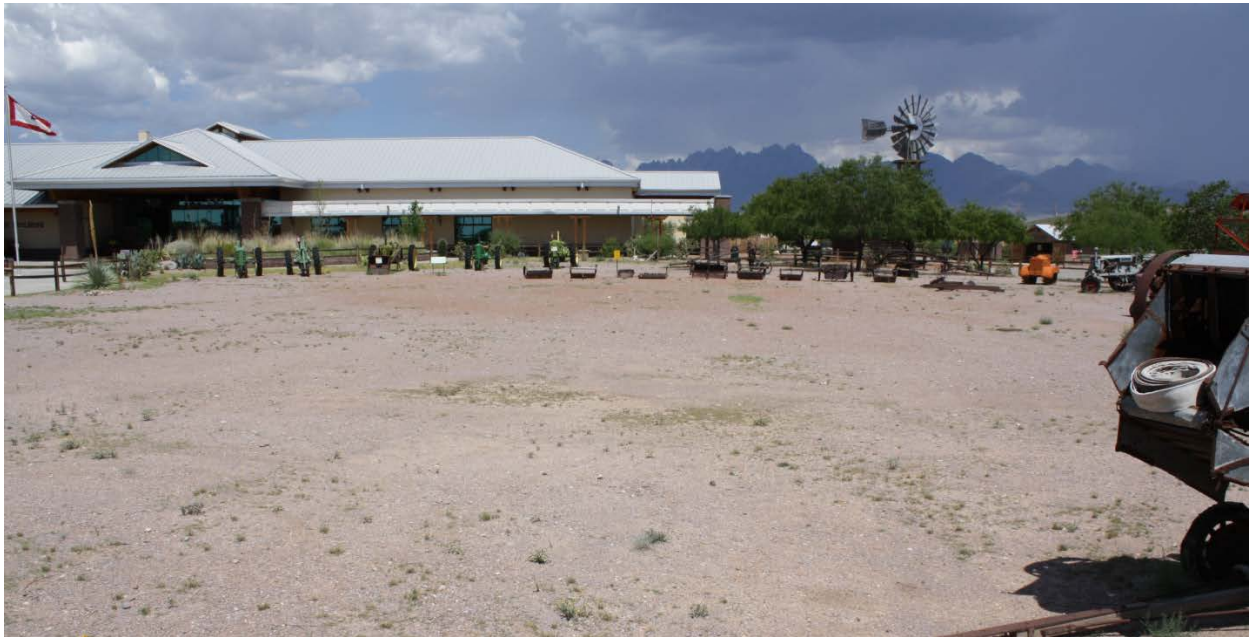
Heritage Garden at Farm Ranch Heritage Museum, before renovations
