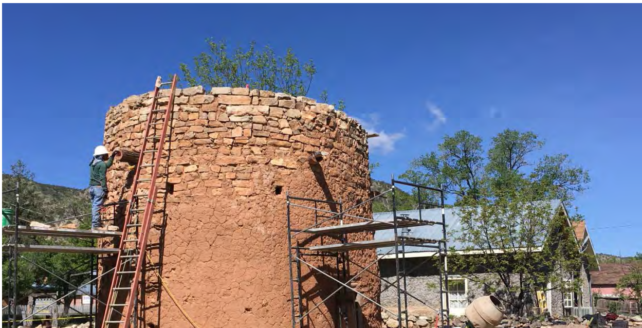
Torreón at Lincoln Historic Site under construction
